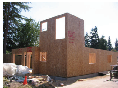
Shelter progress - July 2009
